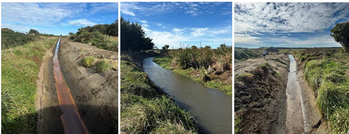
Figure 2: Drains following mechanical clearance
